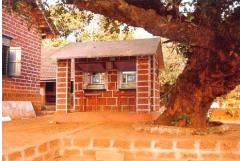
Figure 2: Photo of an MIE kiosk, Sindhudurg
